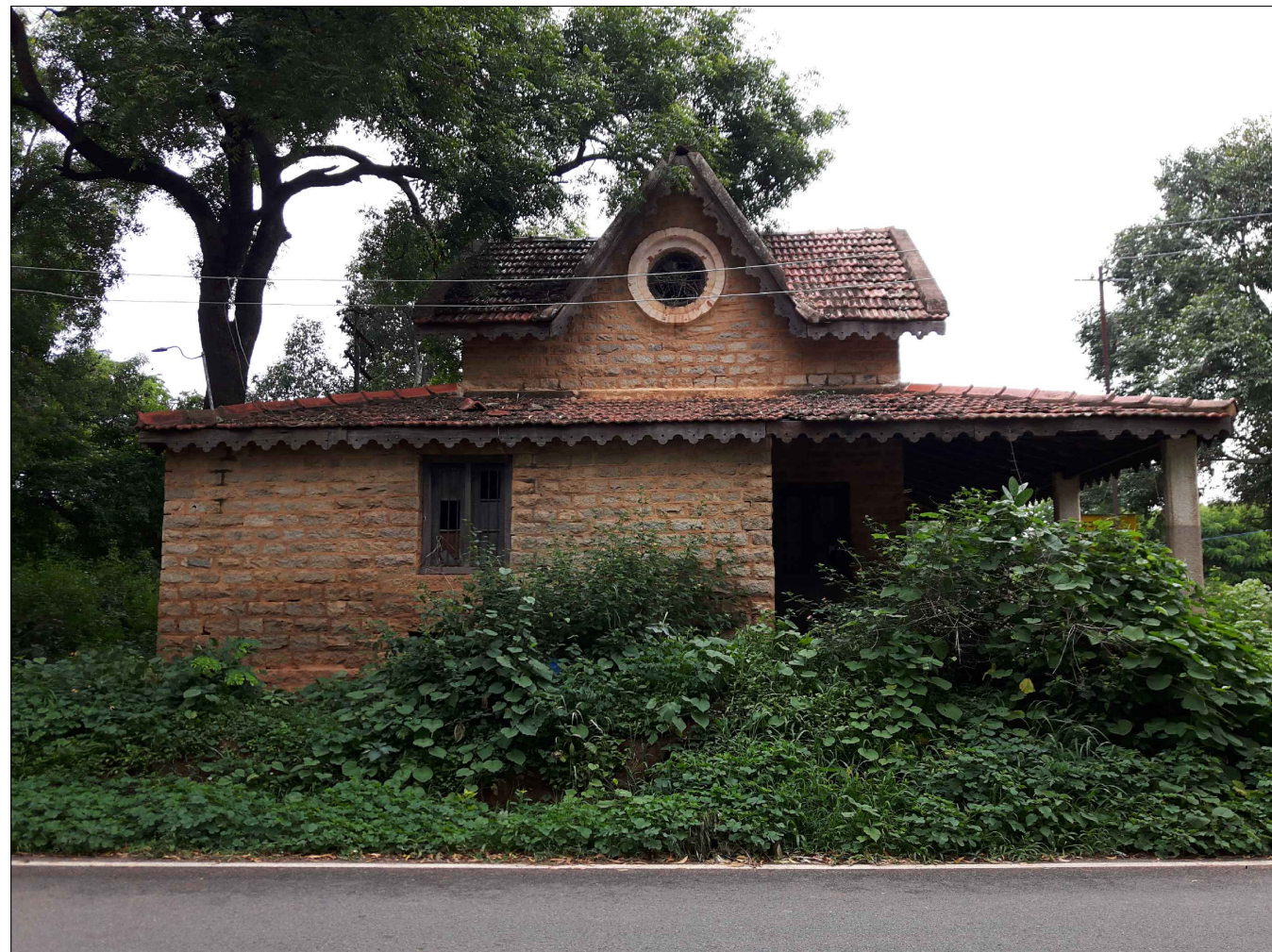
(Source: Photo Taken by Ar. Sharan Desai)
